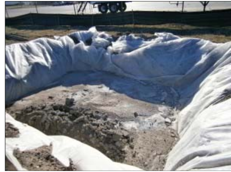
Plate 4.6 Concrete washout area
