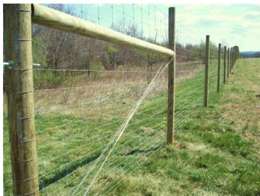
Plate 4.3 – Deer fencing for perimeter fence
