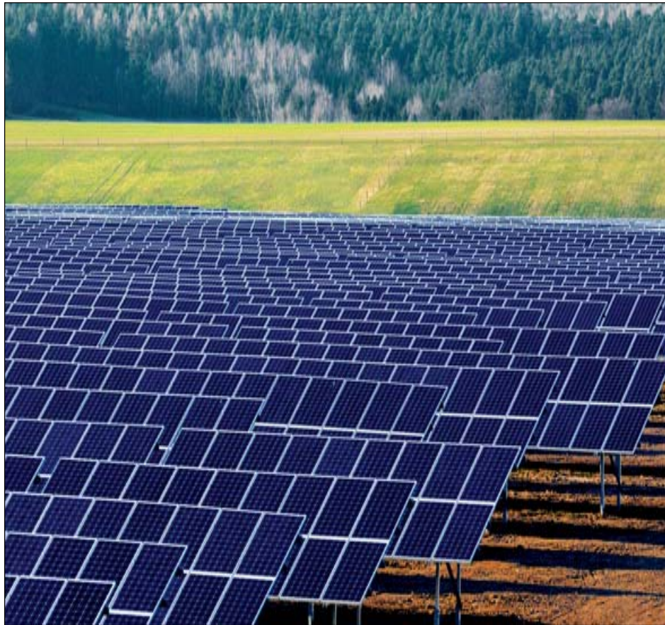
Plate 4.2 Example of a Ground Mounted solar PV array
