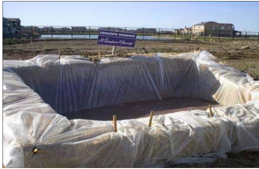
Plate 4.5 Concrete washout area
